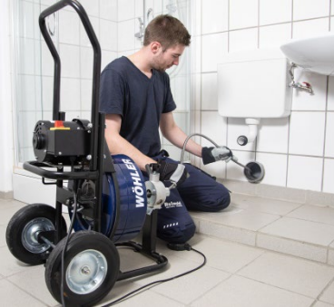
Fig. 7: Drain cleaning
