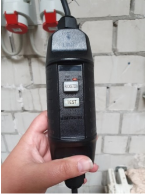
Fig. 6: PRCD-Switch
