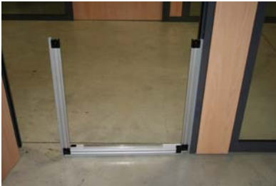
Fig. 11: Assembly of the lateral elements
